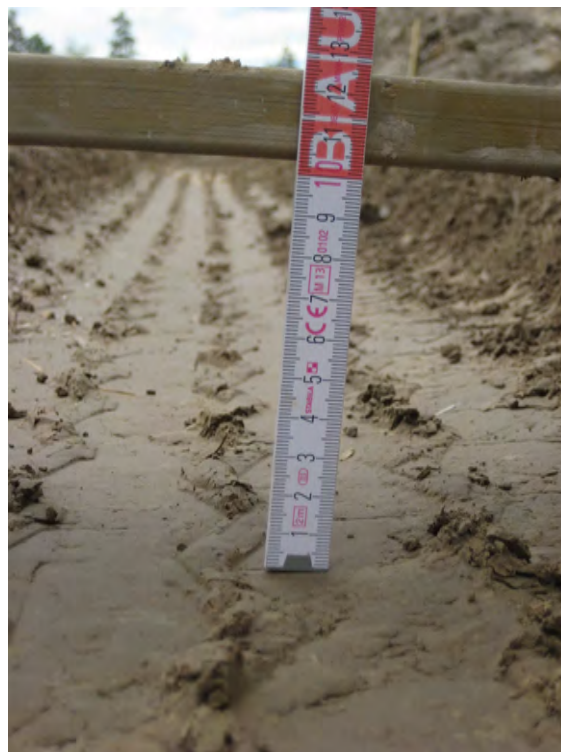
Ruts due to compaction (2015). Picture: T. Seehusen
